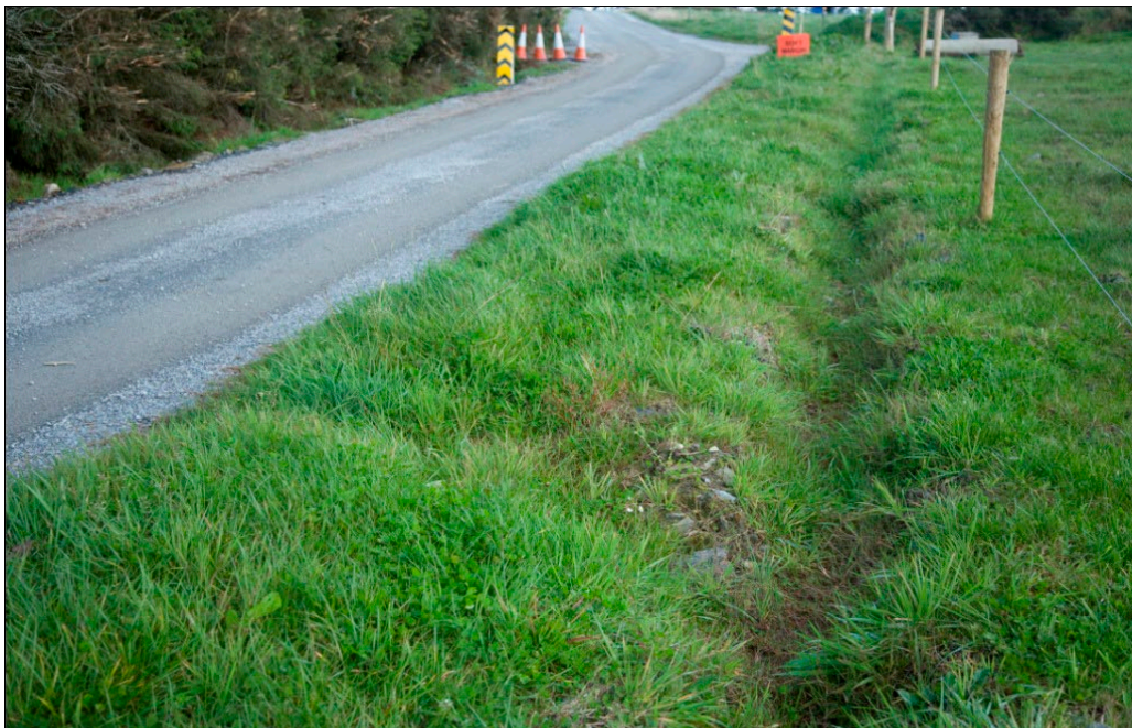
Plate 2-2: Grassed Swale along Access Track
